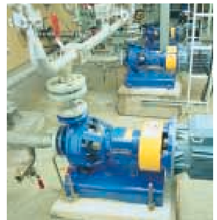
Regarding smaller motors, it is an advantage if the motor is flanged directly against the bearing assembly.
